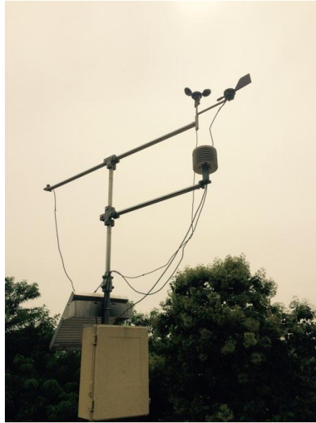
Figure -3.1 Meteorological Monitoring Station Installed
